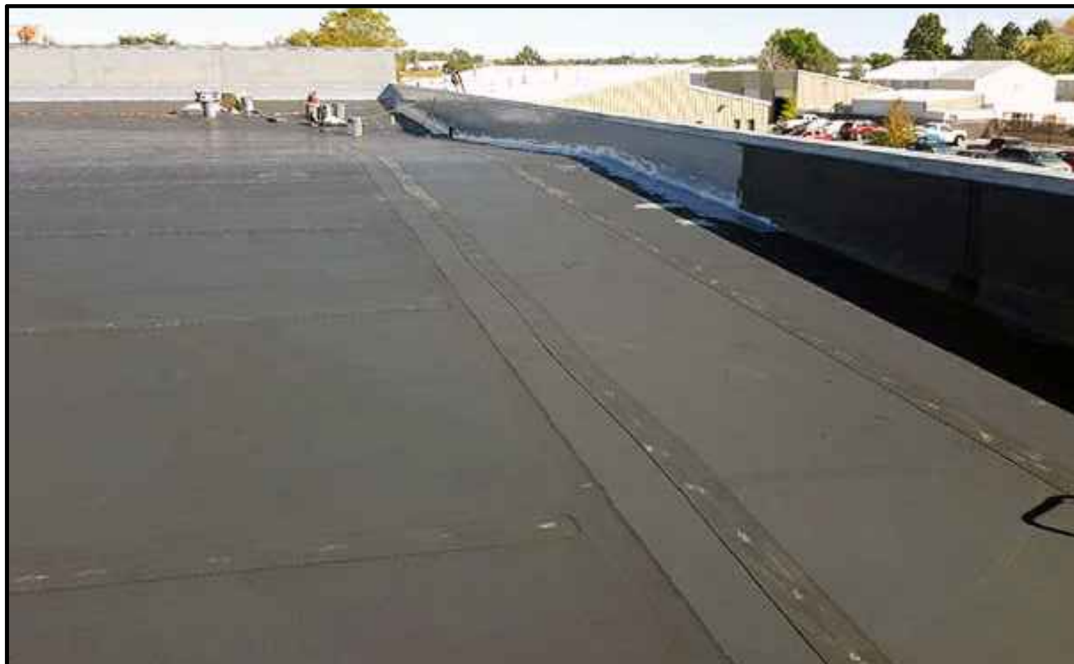
EPDM ROOFING - FIRESTONE FULLY ADHERED BLACK EPDM ROOFING
