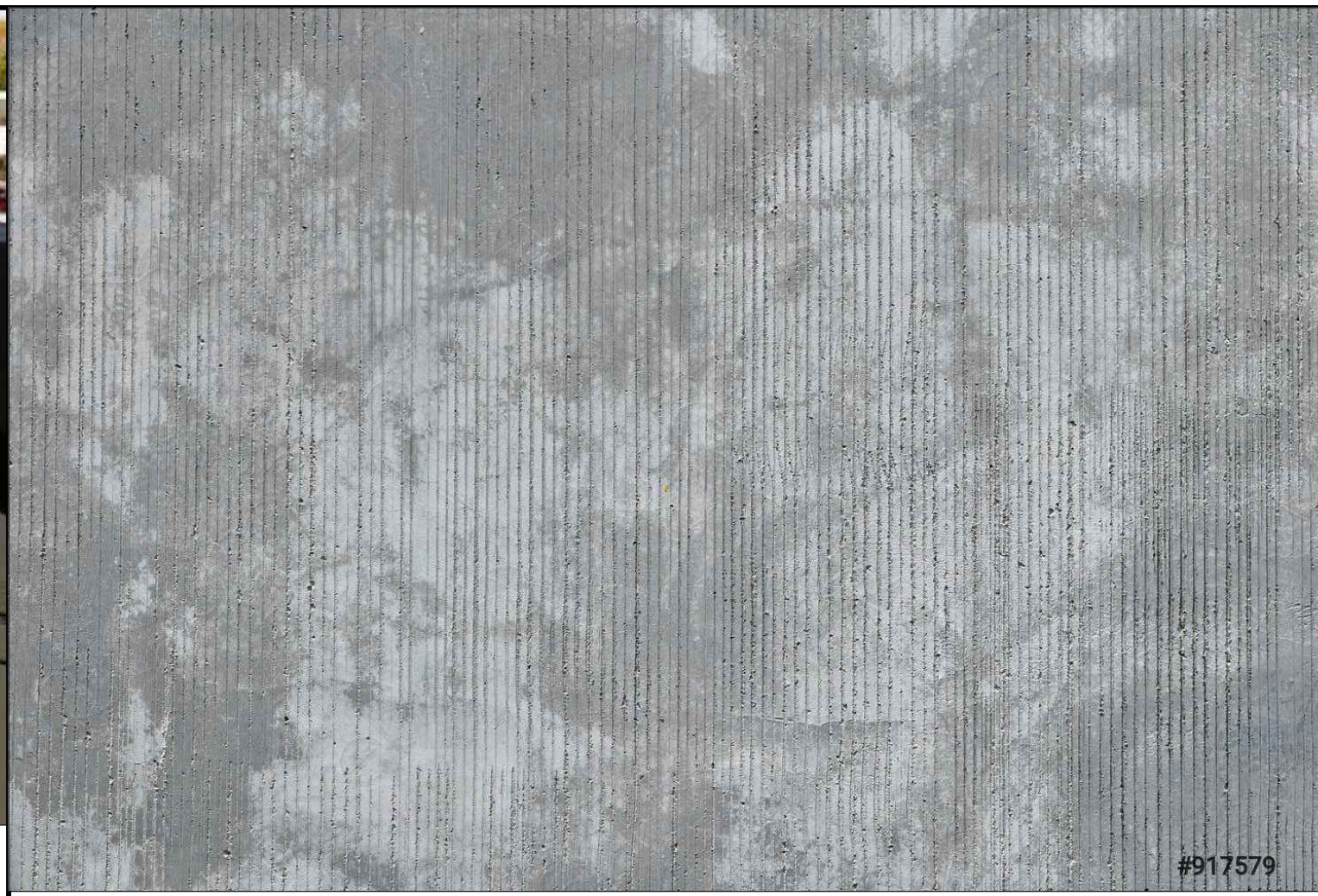
RUBBED CONCRETE FOUNDATION WALL
